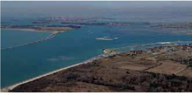
2. Lido inlet. Reinforcement of the south jetty and, on the foreground, the new island
